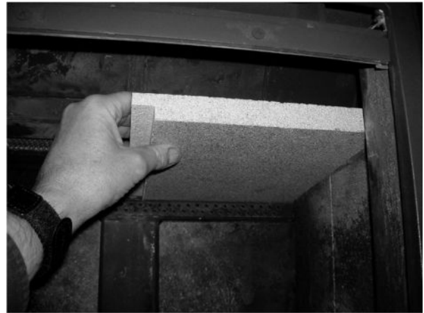
Figure 18 (cont.) - Removing/Replacing the Baffle for Inspection
