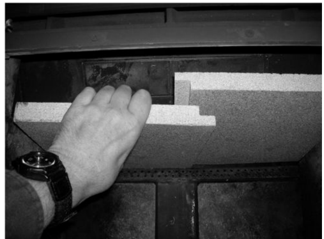
Figure 18 - Removing/Replacing the Baffle for Inspection
