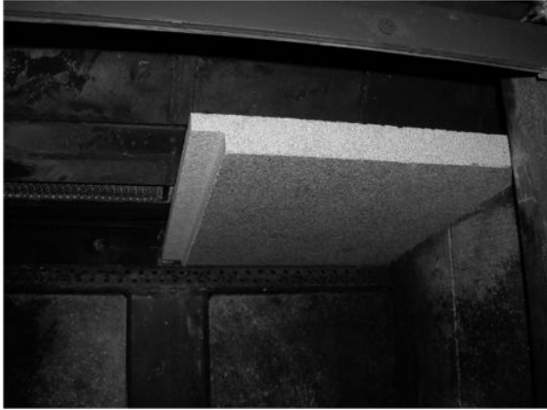
Figure 18 (cont.) - Removing/Replacing the Baffle for Inspection
